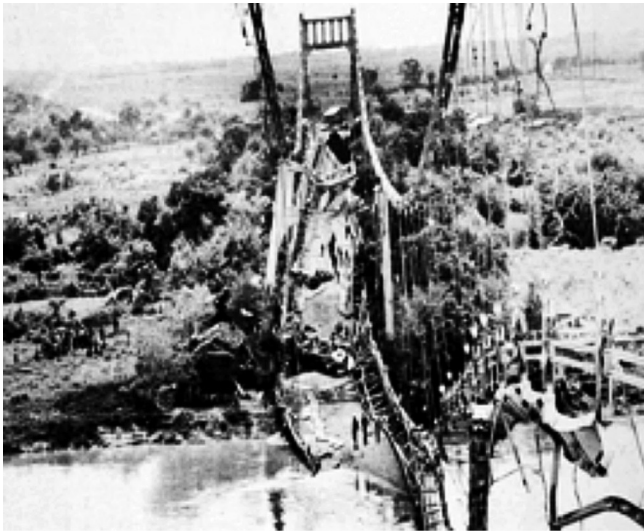
Cuscatlan Bridge over the Pan-American highway, and Golden Bridge on the Littoral highway, before and after the civil war. The Cuscatlán was dynamited on January 1st, 1984, and the Puente de Oro, on October 15, 1981.
